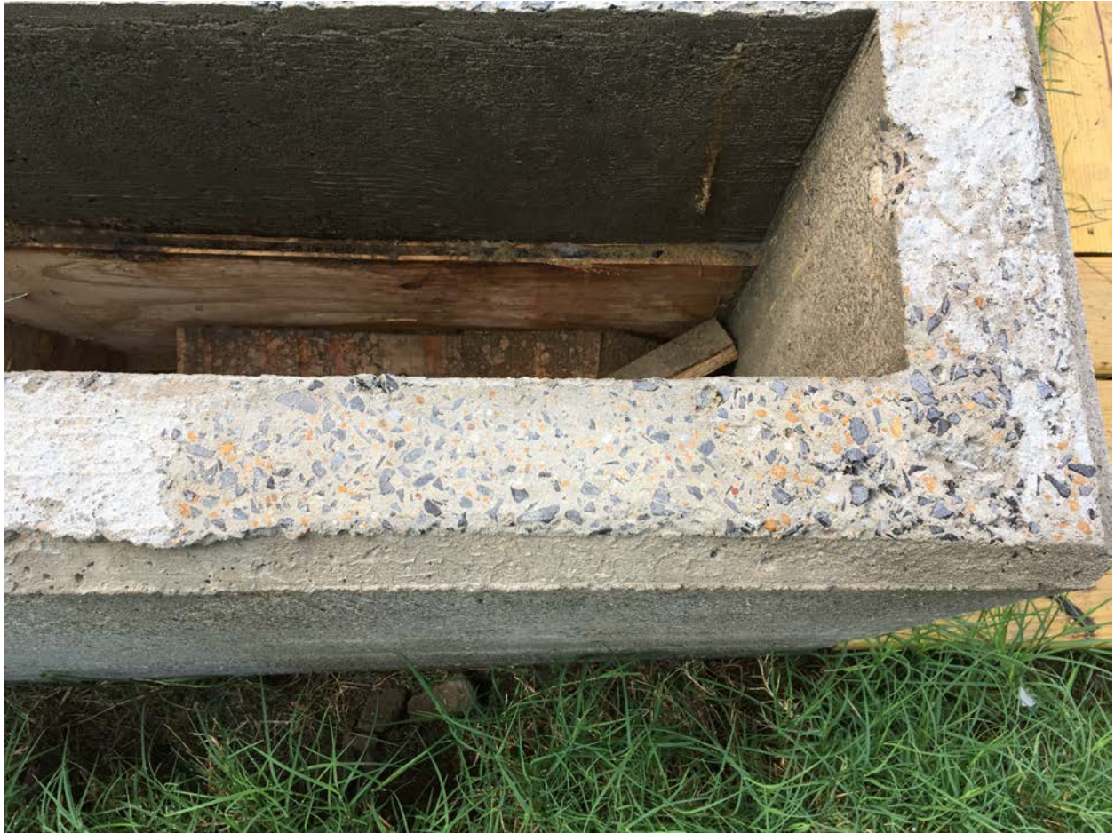
Starting to polish the top band of the concrete.
