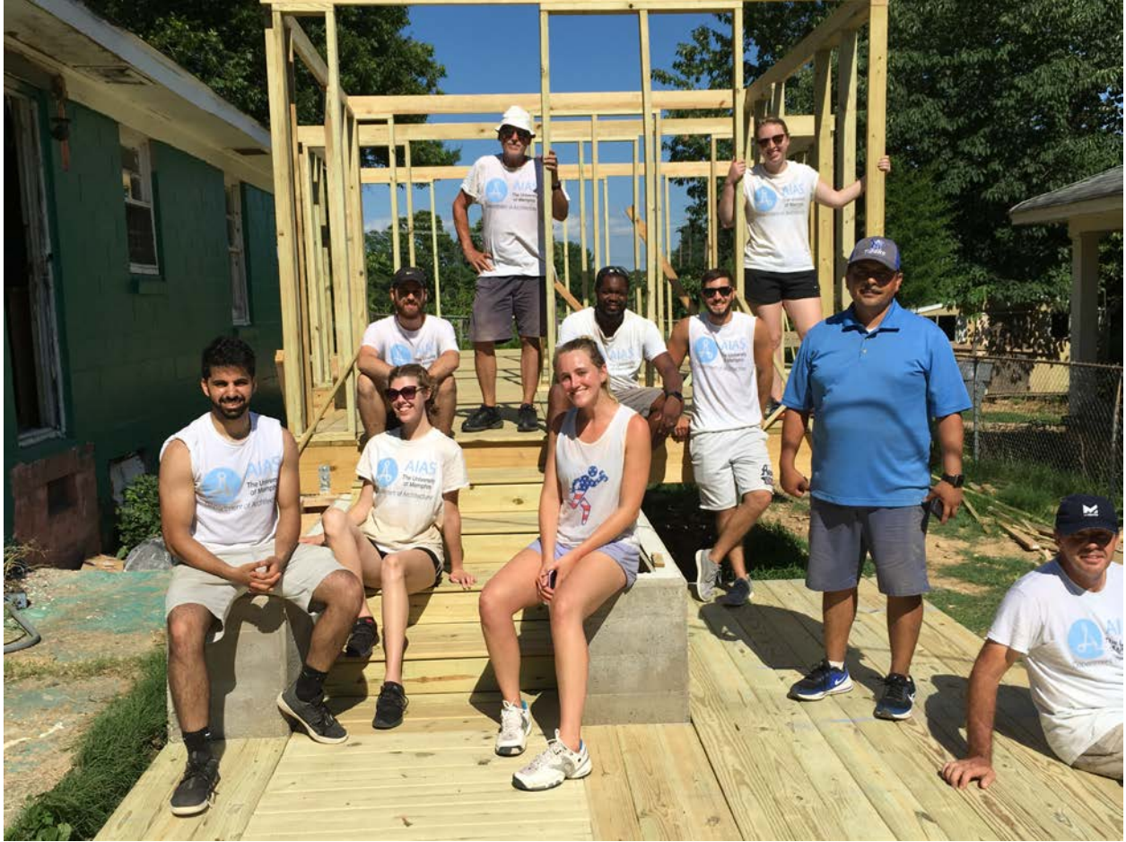
The first module is framed and the “first step” deck is complete!
