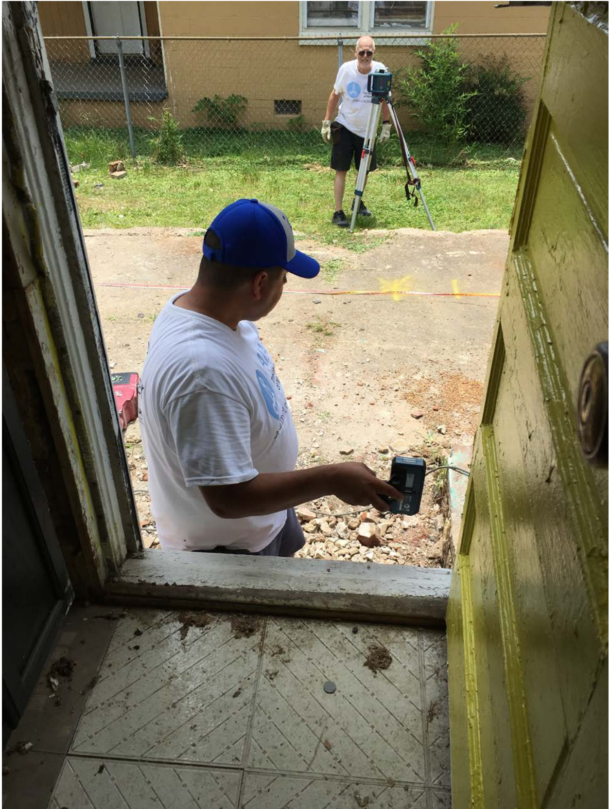
Getting points to ensure the floor of the house is level to the floor of the outdoor rooms.
