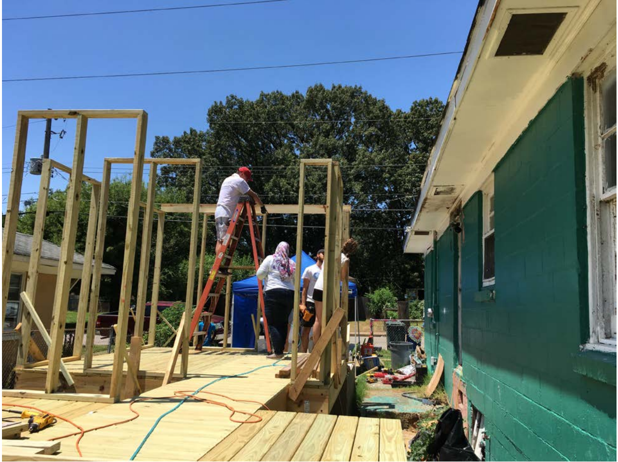
The framing for the walls starts.
