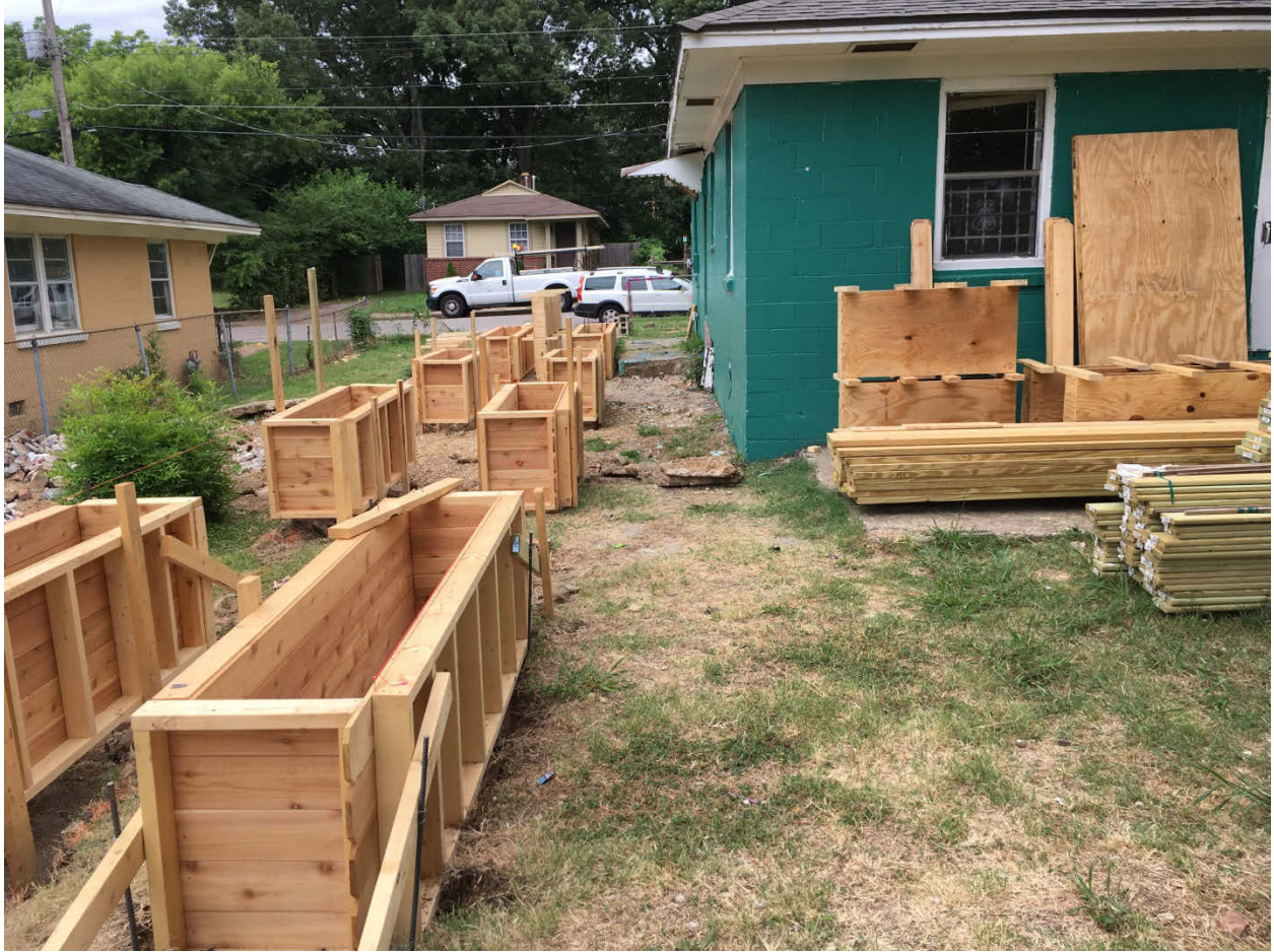
Exterior forms almost all in place. Internal forms stacked against the house.
