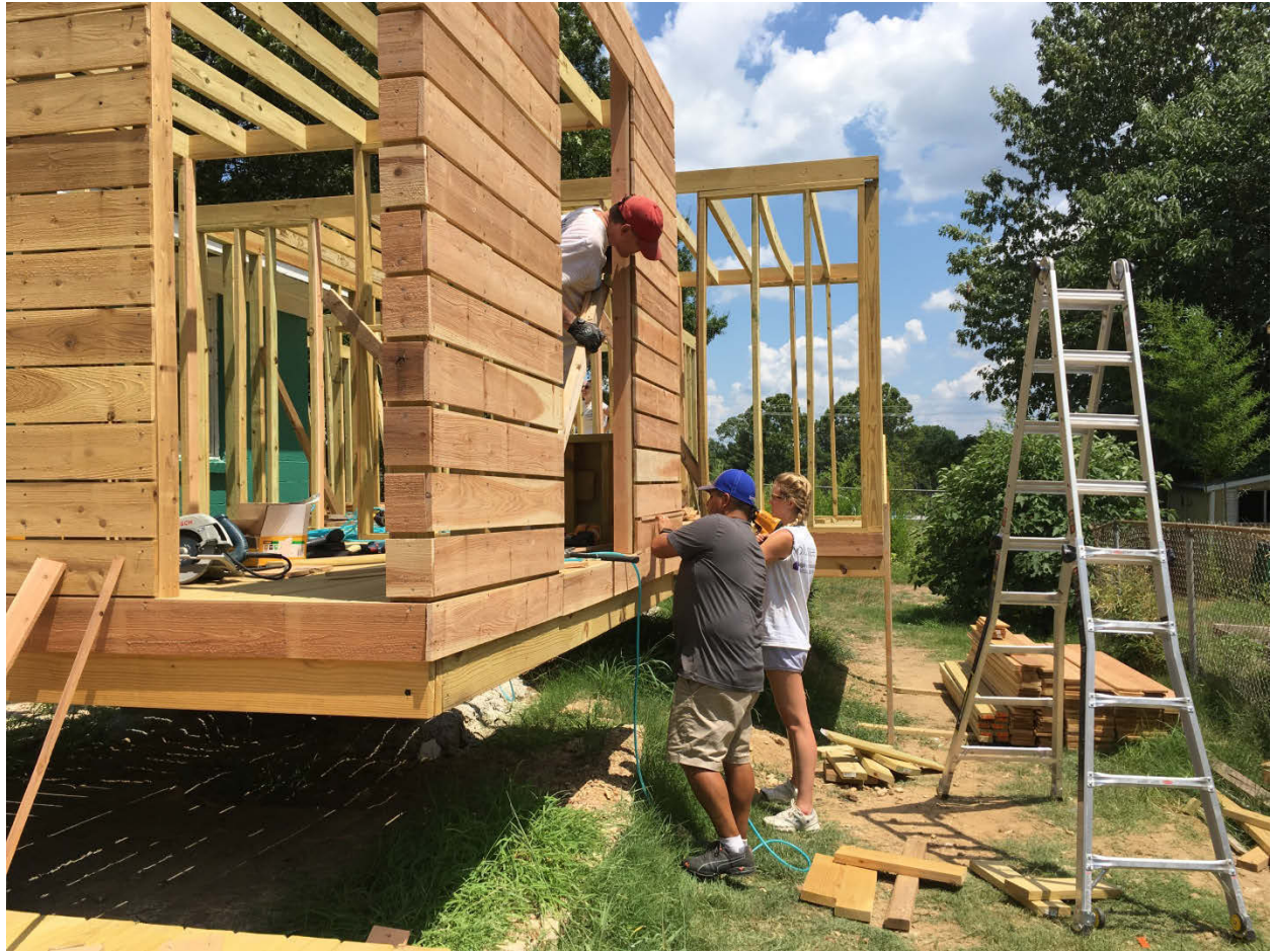
The installation of the cedar cladding is well underway.
