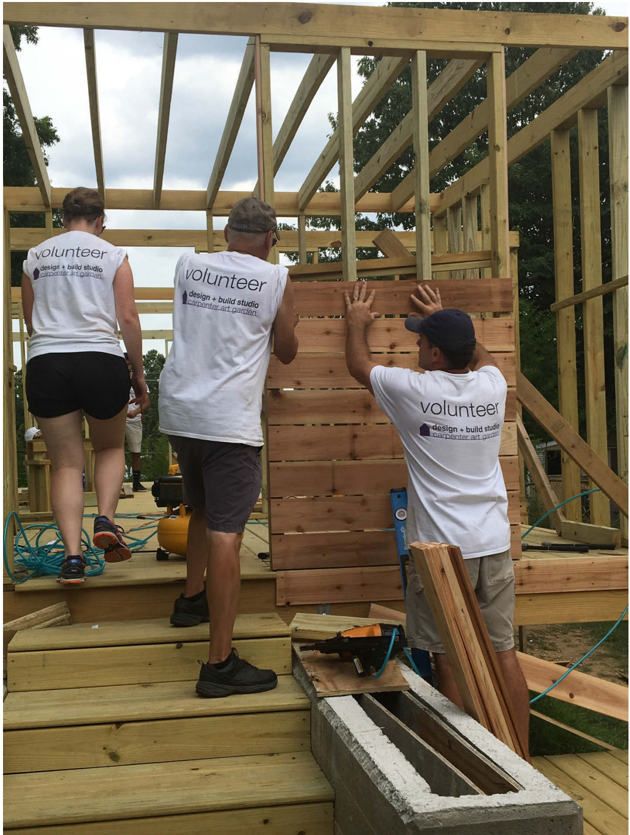
The cedar cladding starts to be put into place.
