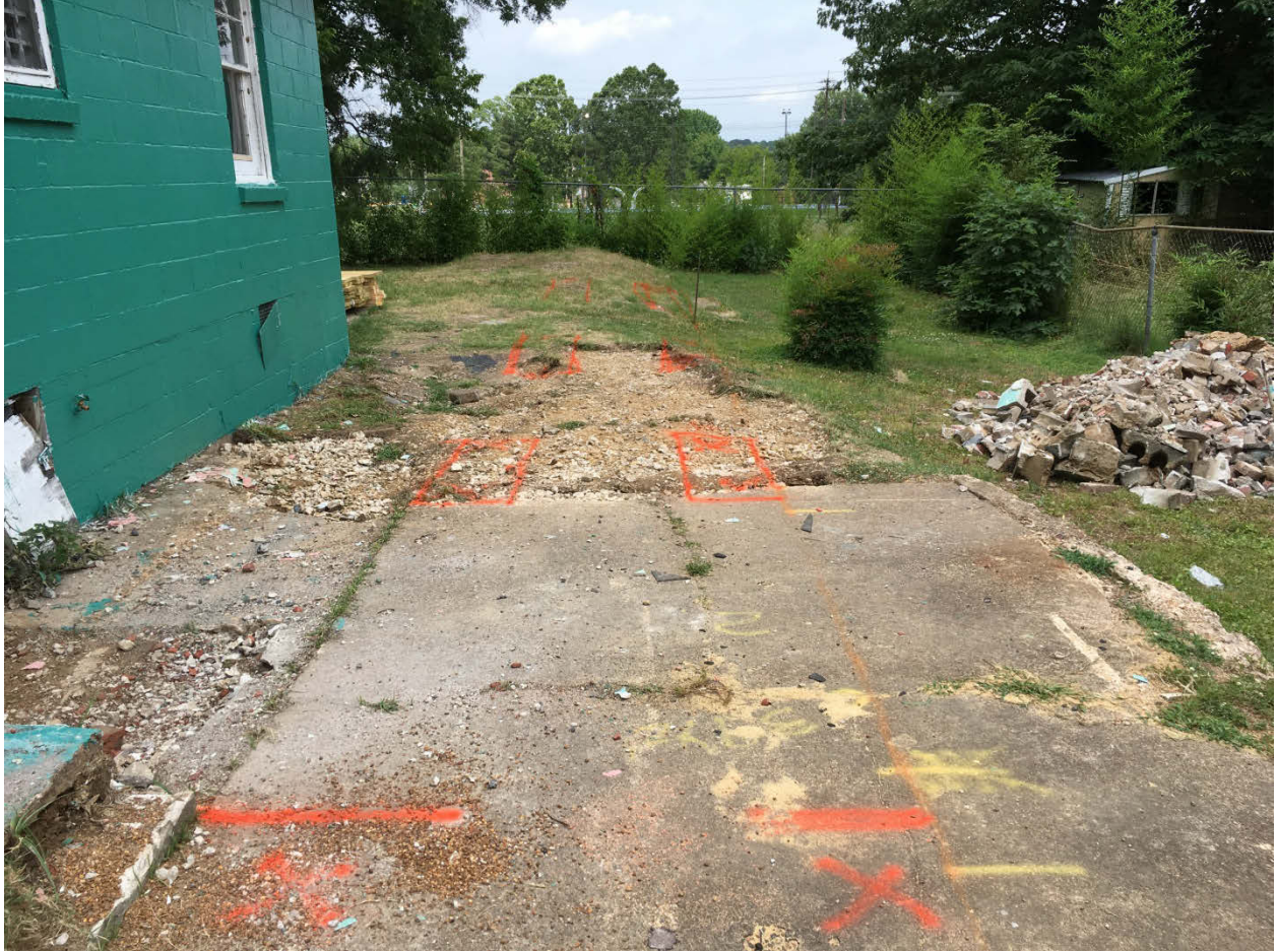
Marking the location of the eight board-formed concrete planter boxes / structural supports.
