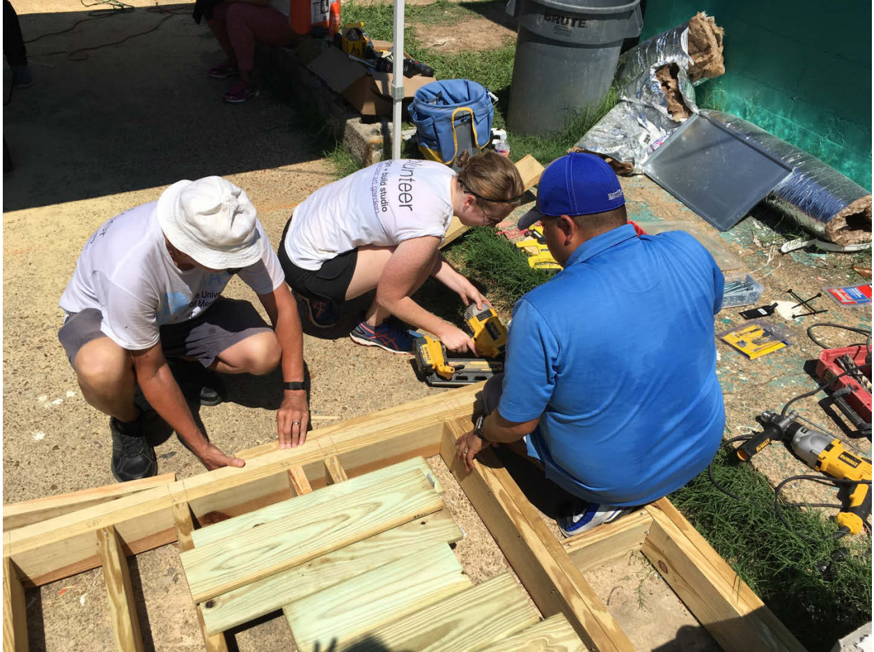
Working on the entry deck.
