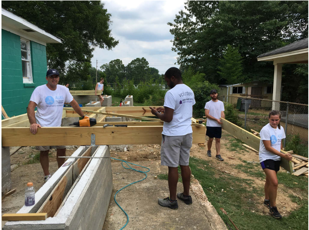
Starting the construction of the outdoor rooms.
