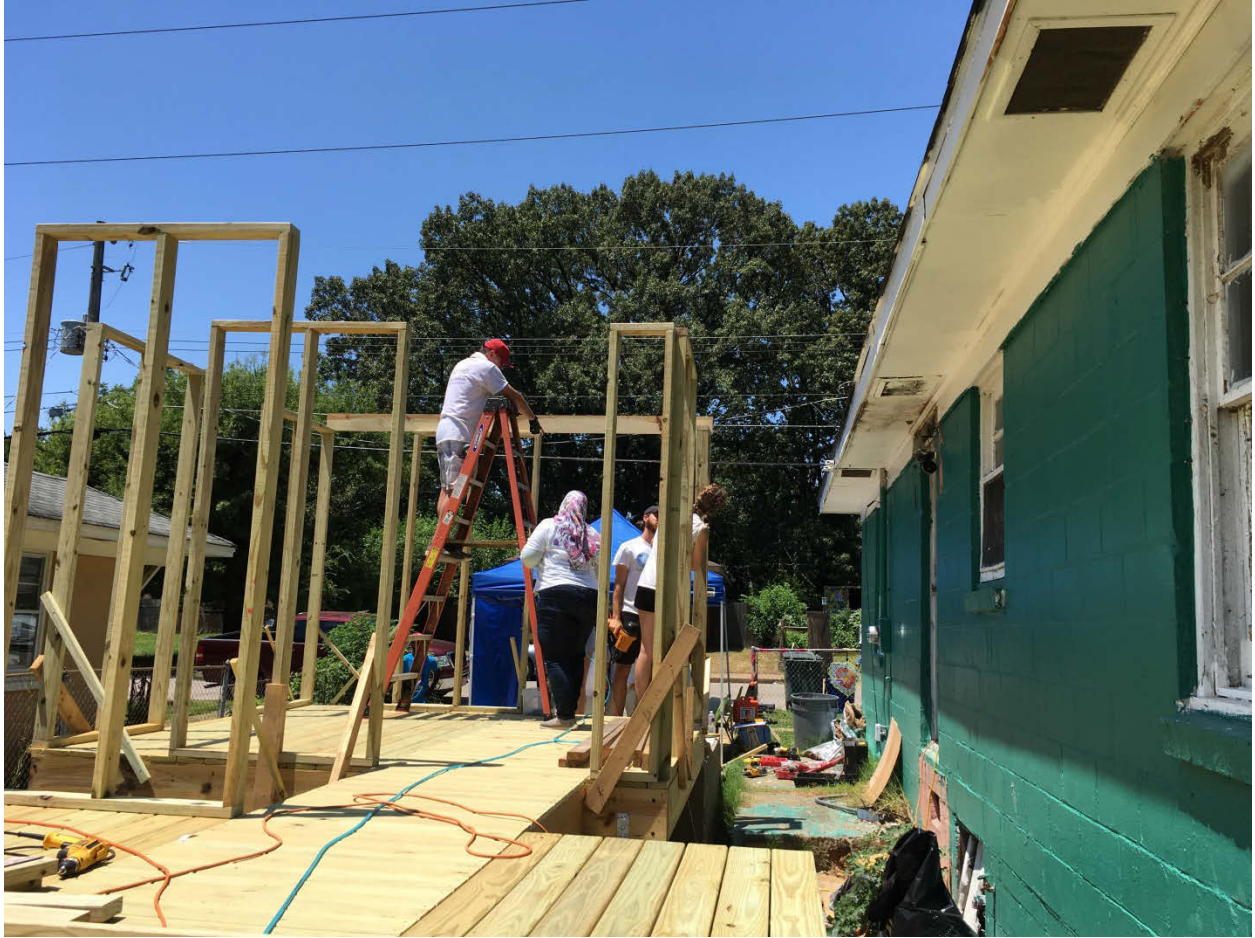
The framing for the walls starts.
