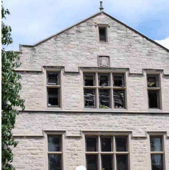
Exterior view of explosion aftermath at Mizzou. Broken windows and mangled interior are visible on upper floor. (Photo courtesy of Columbia Missouri Fire Department.)
