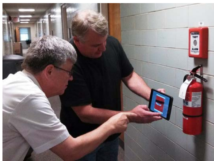
Tom Eadie (I) demonstrates the finer points of scanning a fire extinguisher barcode with the iPad Mini
