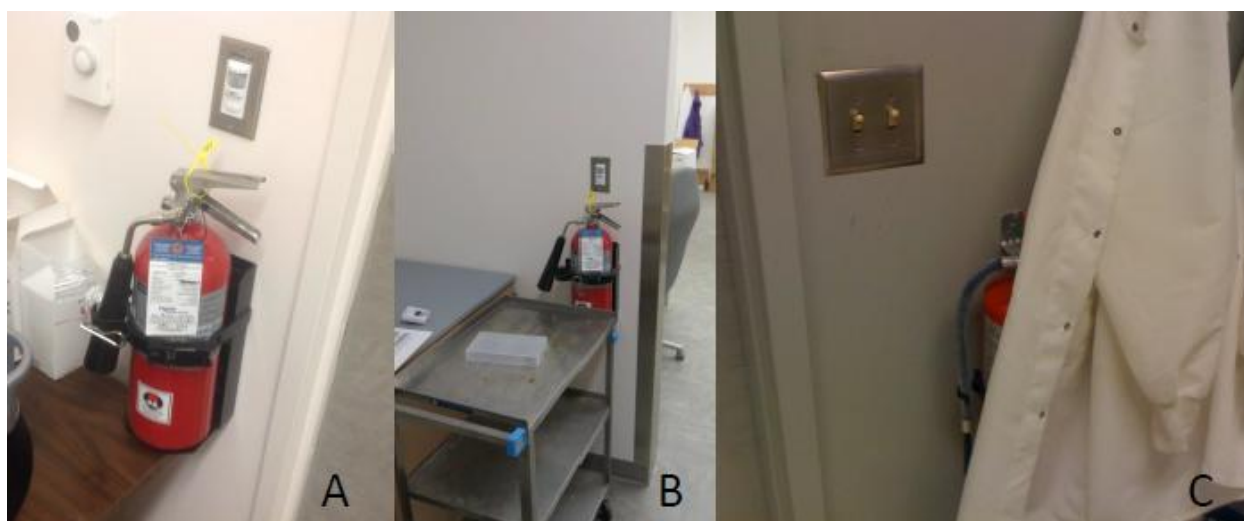
Figure 15: Fire Extinguishers. A-Accessible fire extinguisher. This fire extinguisher is free of obstructions and plainly visible. B-Obstructed fire extinguisher. A cart is blocking this extinguisher; this would be considered a safety violation. C-Hidden fire extinguisher. It is important to make sure fire extinguishers are not only unobstructed, but also clearly visible. While this extinguisher is accessible, it is not easily seen.
