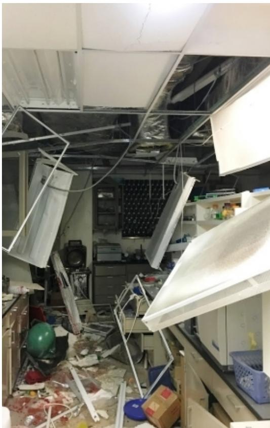
Honolulu Fire Department photo shows damage resulting from explosion of a pressure vessel
