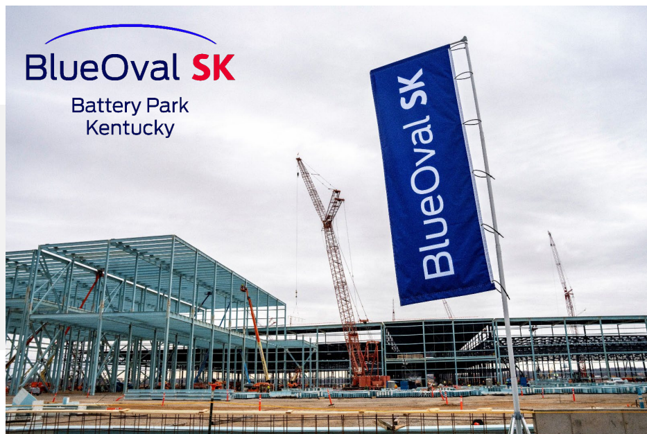
BlueOval SK Battery Park – Glendale, Kentucky
